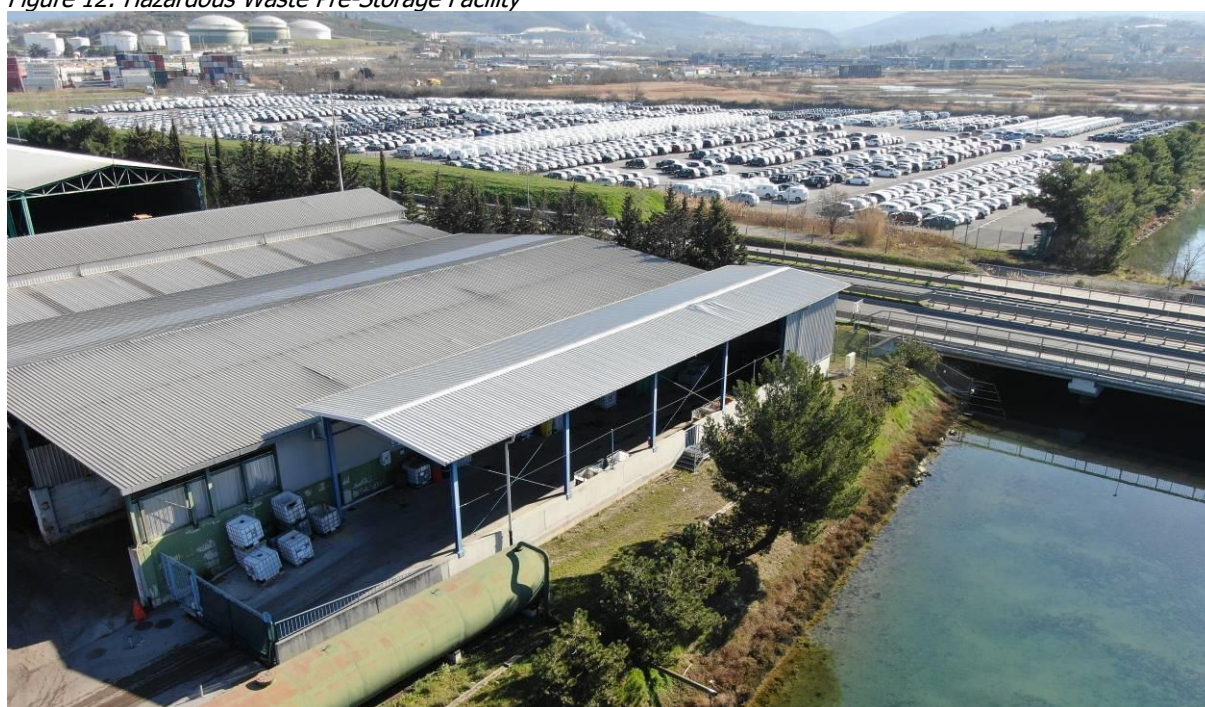
Figure 12: Hazardous Waste Pre-Storage Facility
