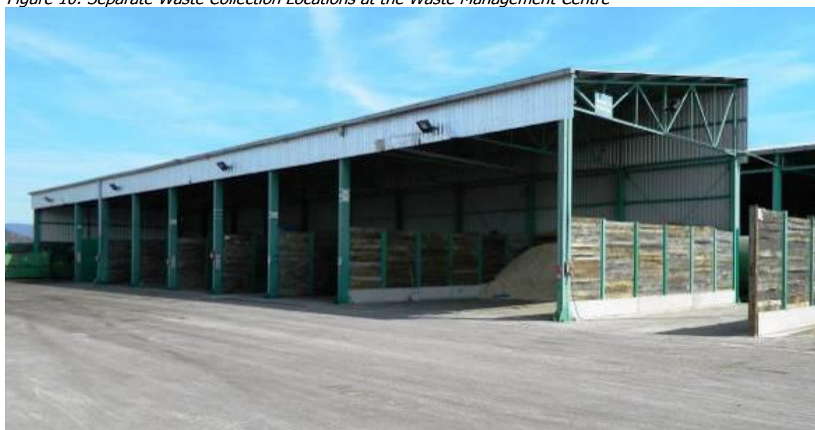
Figure 10: Separate Waste Collection Locations at the Waste Management Centre
